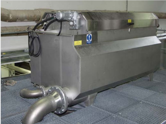
Stand alone MDF with inlet and outlet flanges
