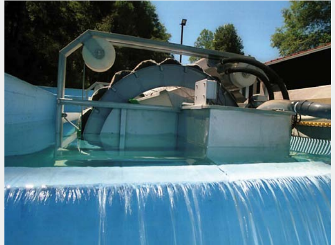
Small channel installation of a domestic STP
